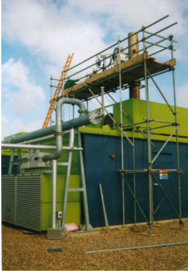
FIGURE 3. SAMPLING PLATFORM INSTALLED ACROSS A CONTAINERISED GENERATING SET, AND CLOSE-UP OF PARTICULATE SAMPLING EQUIPMENT INSTALLED ON SCAFFOLDING
