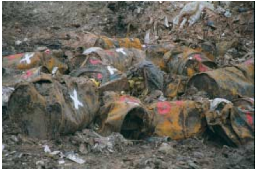
Re-excavated drums of industrial waste awaiting consignment to a special waste landfill
