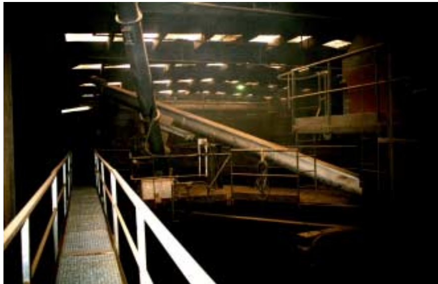
Sawdust and solvent mixing treatment facility, Sobry treatment plant, Roeselare, Belgium
